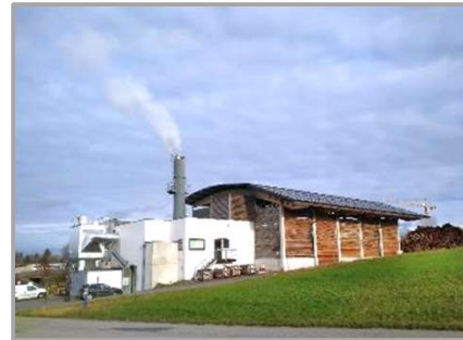
Seekirchen, 2022 Heat recovery 500 kW
