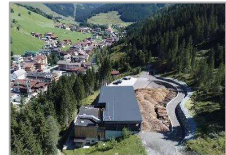
Gerlos, 2023 Heat recovery 740 kW
